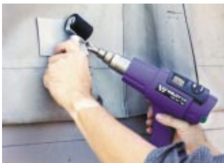
Repairing a tarpaulin by welding on a patch.
