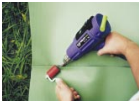
Welding a Biotope film made of PVC.
