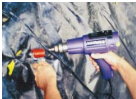
Welding a damaged PVC cover.
