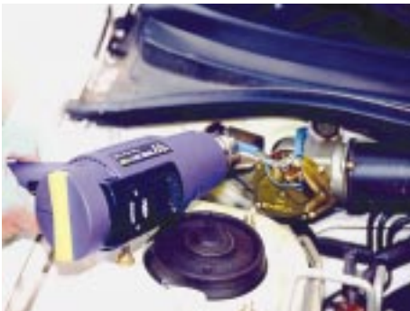
Shrinking a PVC heat-shrink tube.
